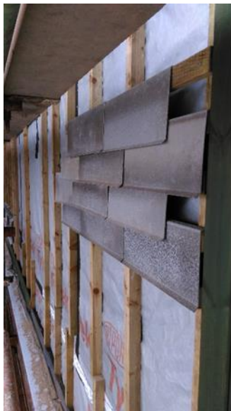
Figure 11 Reused aluminium for external wall cladding
