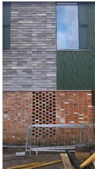
Figure 11 Reused aluminium for external wall cladding
