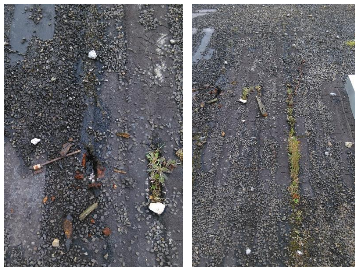
Figure 12 - Damaged roof board
