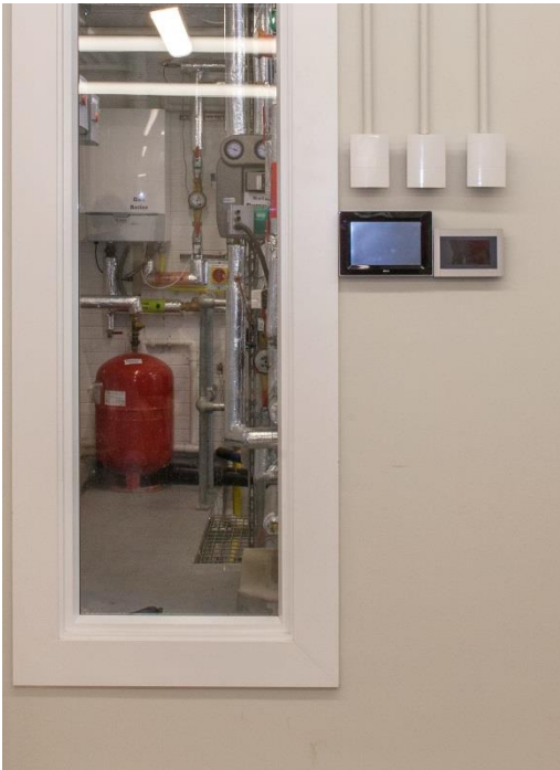
A look into the Plant room and the CHP system located in every room.
